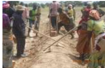
NR: Soil compaction with compactor
