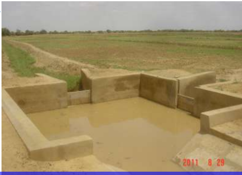
Repairing the distributor
