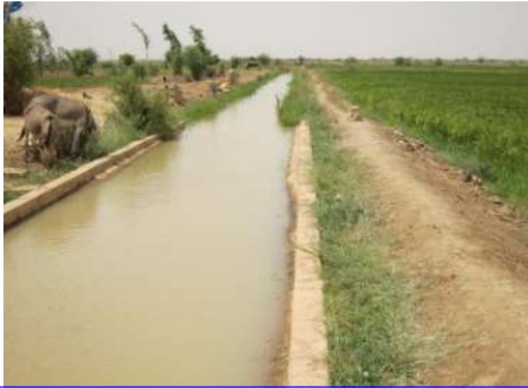
Repairing the main canal
