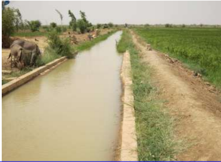
Repair of the main canal
