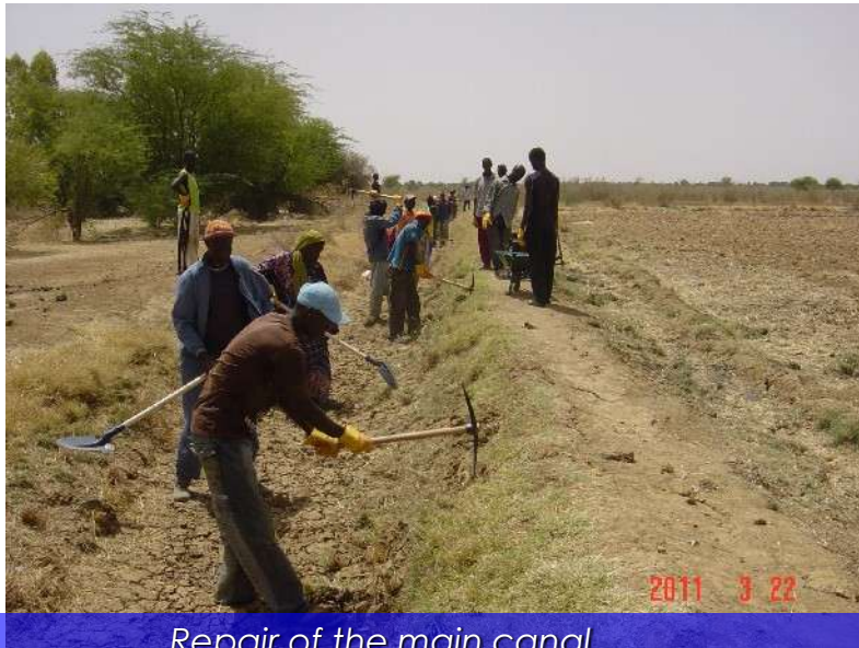
Repair of the main canal
