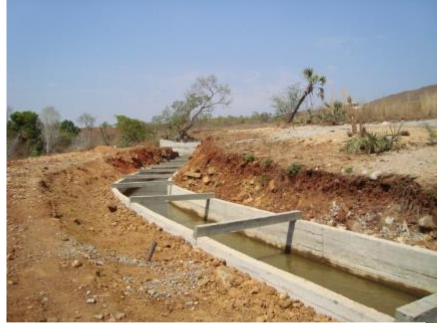
Concrete work of main canal
