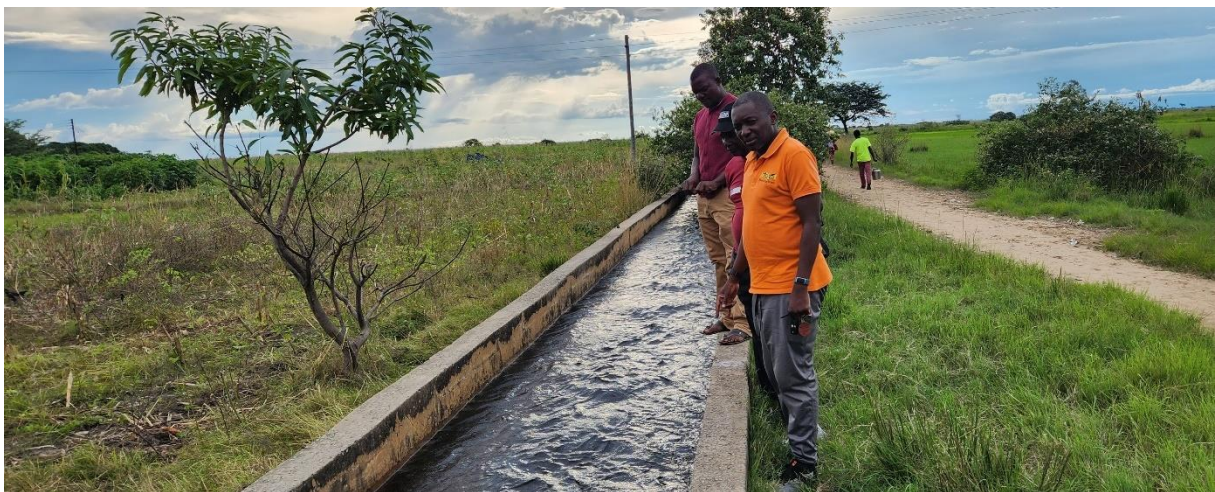
Figure 9-10: Inspection of the Sefula Irrigation Scheme Water Canals
